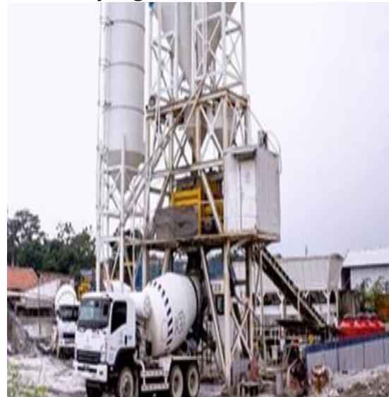
Gambar 7 Batching Plant Proyek
