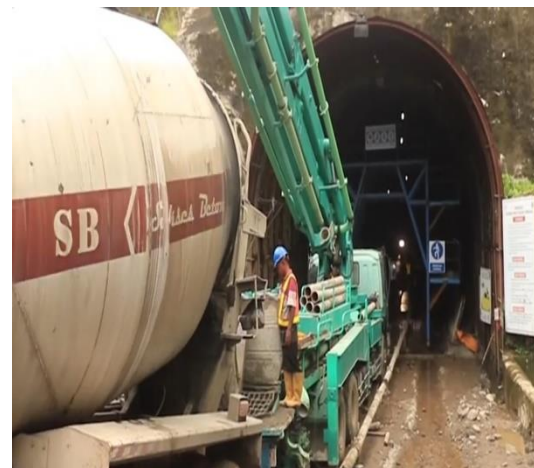
Gambar 2 Foto Proses Muat Beton ke Concrete Pump
