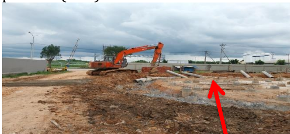
Gambar 5: Cutting Pile
