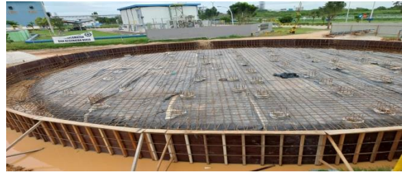
Gambar 7: Pembesian Pondasi Tangki
