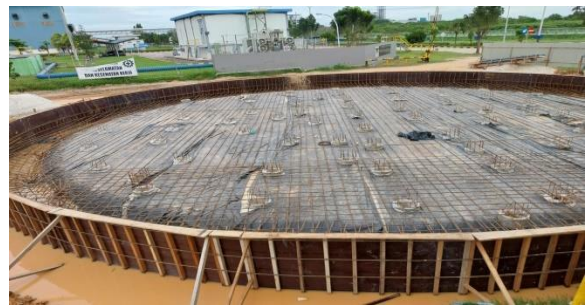
Gambar 7: Pembesian Pondasi Tangki
