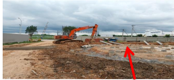
Gambar 5: Cutting Pile
